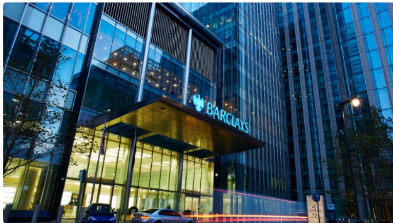
Barclays Head Office at 1 Churchill Place
